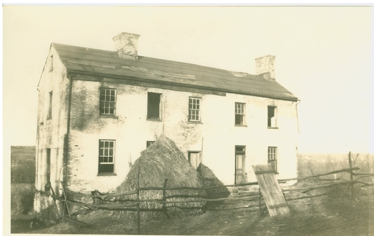
A photograph of Carlyle’s Torthorwald, in 1937, prior to the Fairlington Construction.
